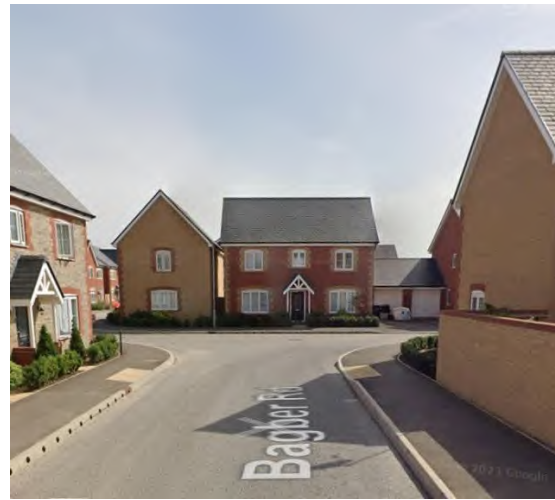
Completed development - Bagber Rd, Stalbridge
