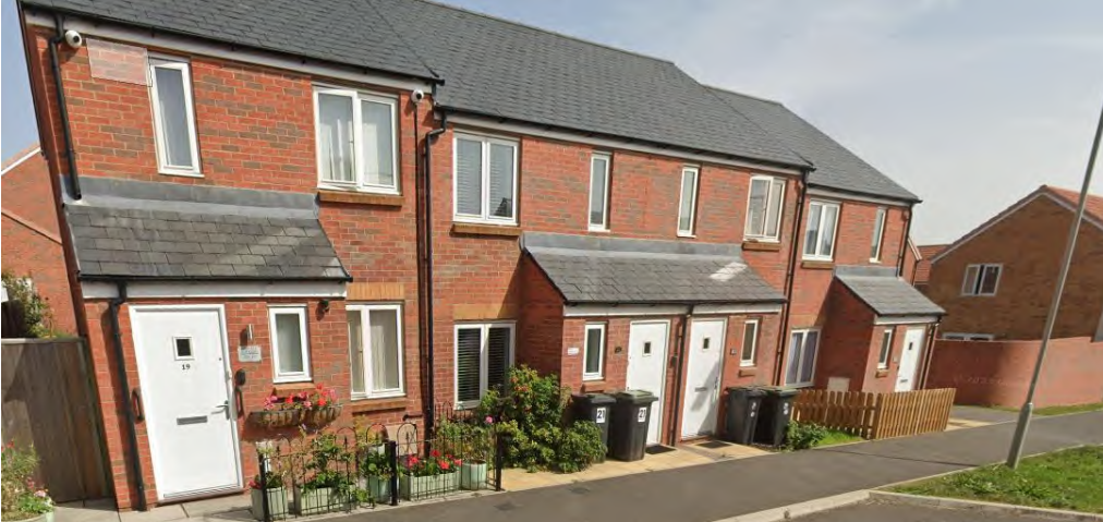
Lack of front boundaries creates opportunities for inconsistency within the street Persimmon – Barton Farm, Sherborne
