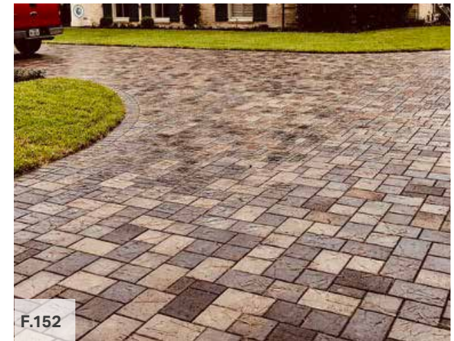
Figure 152: A good example of permeable paver (Source: https://www.paverconnection.com/testimonial/hedwig-village-permeable-driveway-and-patio-upgrade/ )
