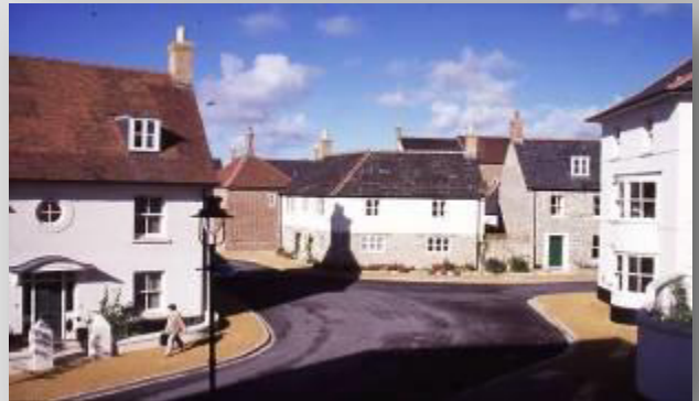
Phase 2 A-D - Netherton Street
