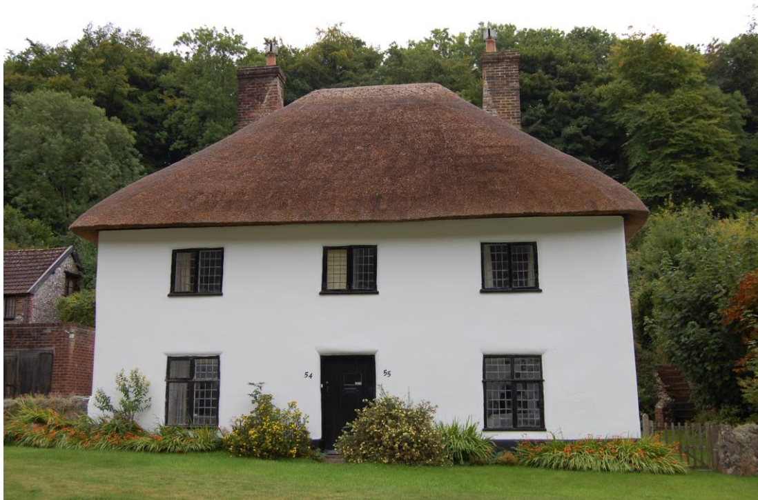
A statutory listed building in The Street
