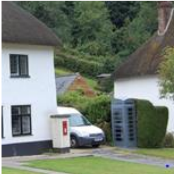
K6 Telephone box adjacent to the Post Office
