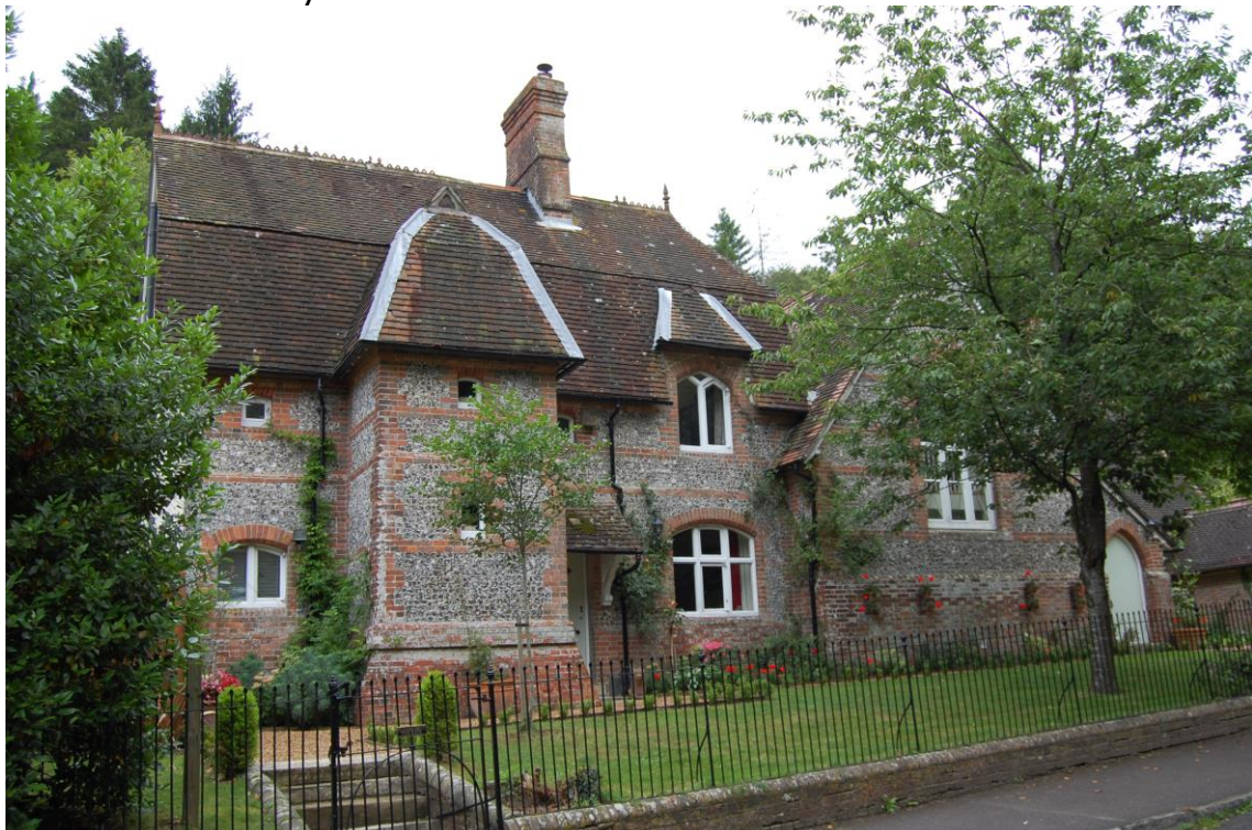
The former Village School and School House
