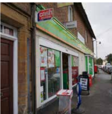
The village shop sits flush to the back of the footway within a mix of residential and business units and is distinguished by the large display windows.
