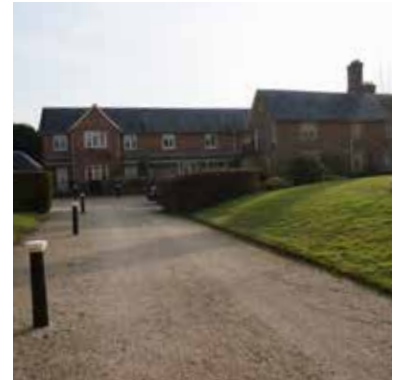
The use of permeable ground materials softens appearances and assists with the control of rainwater run-off.
