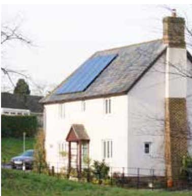
Careful orientation of buildings and the pitch of roofs can allow for the capture of solar energy. Panels can be easily fitted to both new and existing properties.
