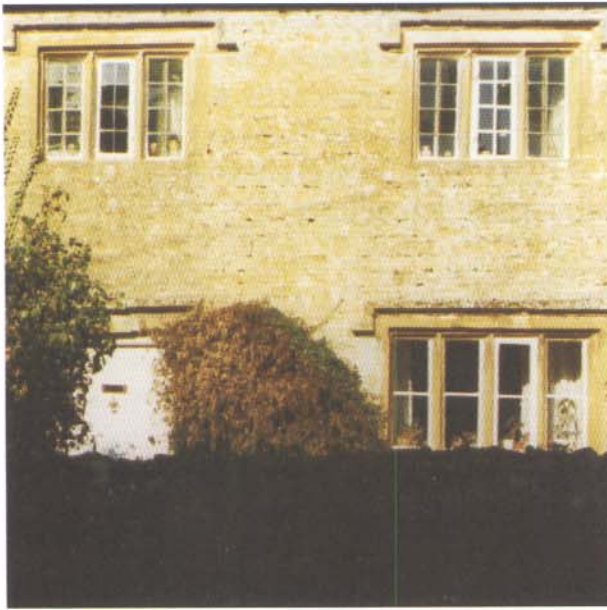
An example of the distinctive mullioned windows, Typical of older Dorset housing
