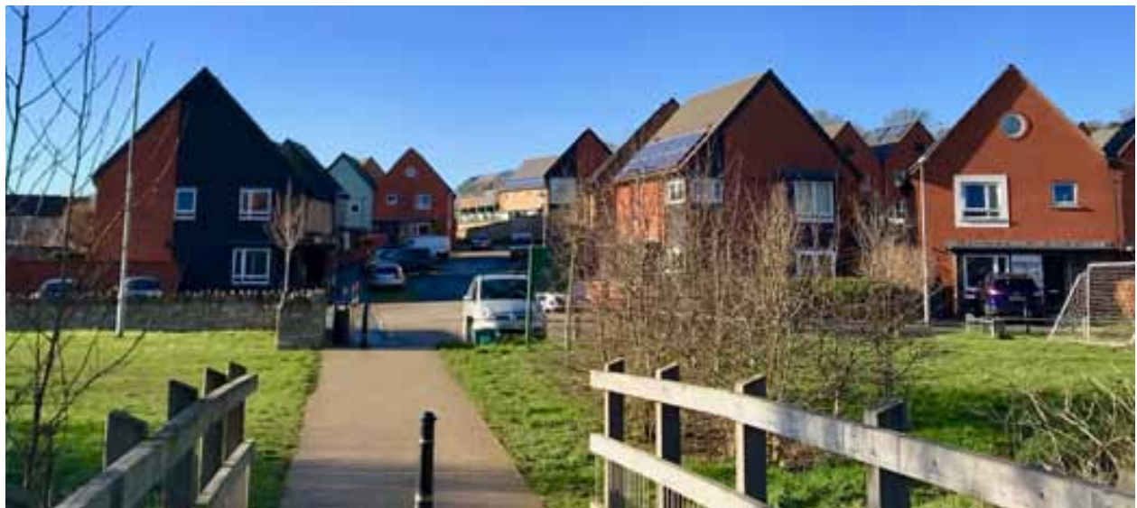
Dibden View, showing Eco Homes
