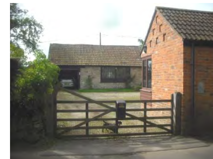
Fig 24 Former blacksmith's (at back) at Edington House
