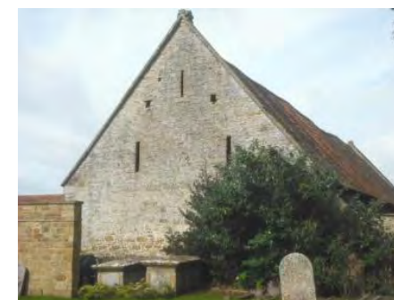
Fig 23 Church Farm's C18 barn as seen from the churchyard
