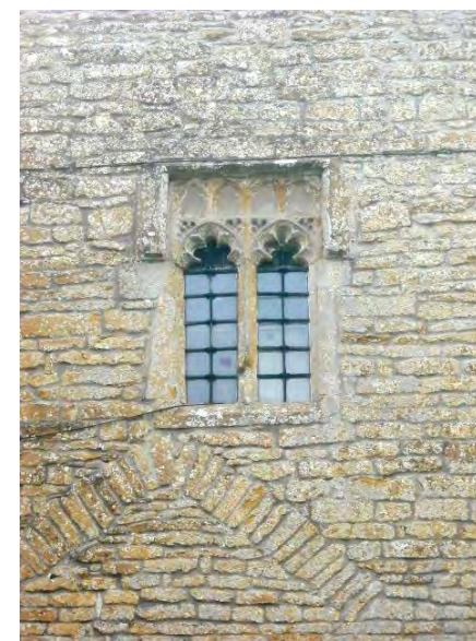
Fig 33 C15 window in NW wall of the Dairy House
