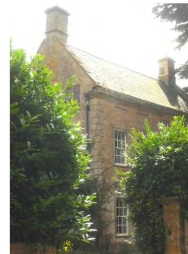
Fig 4 West side of The Rectory
