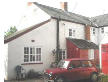
Fig 22 No 20 with the former post office/shop lean-to premises
