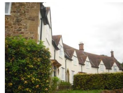
Fig 28 Nos 1-6 Rigg Lane Cottages
