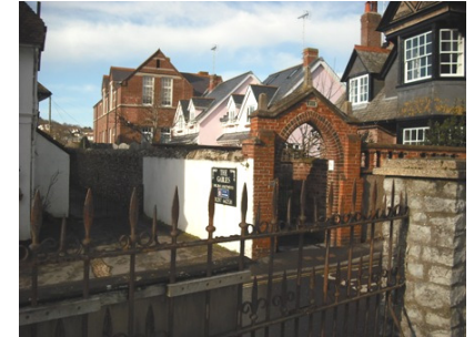
Fig 39 Former primary school
