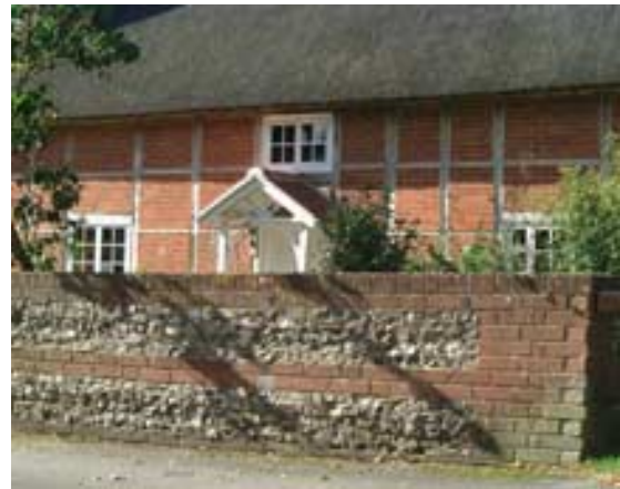
Flint and brick boundary wall to Elm Tree Cottage
