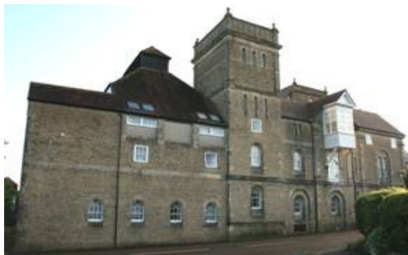
Figure 13: The former Wyke Brewery, Wyke Road.
