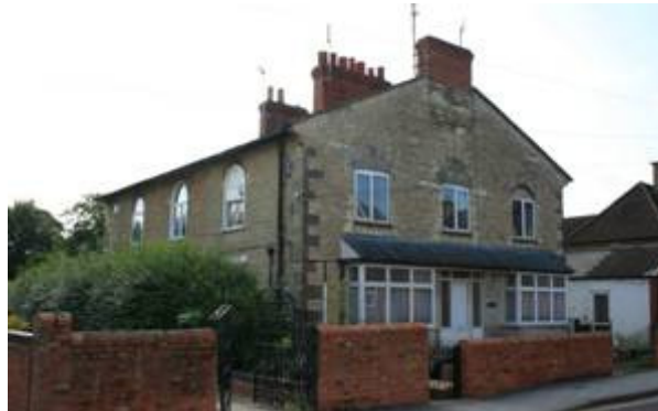
Figure 14: The old Wesleyan Methodist Chapel, Portland Cottages, Queen Street.
