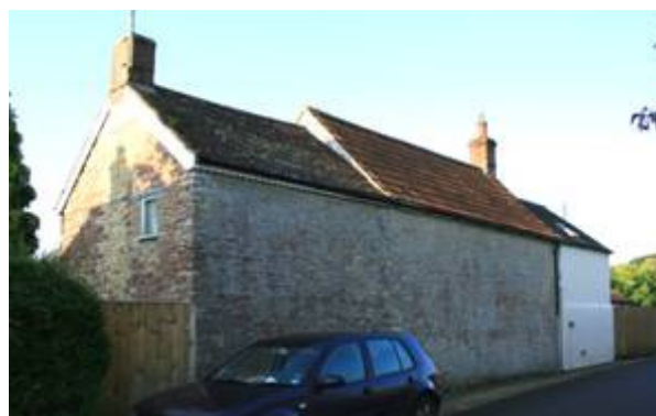
Figure 19: Thistledown Cottage, Wavering Lane West.
