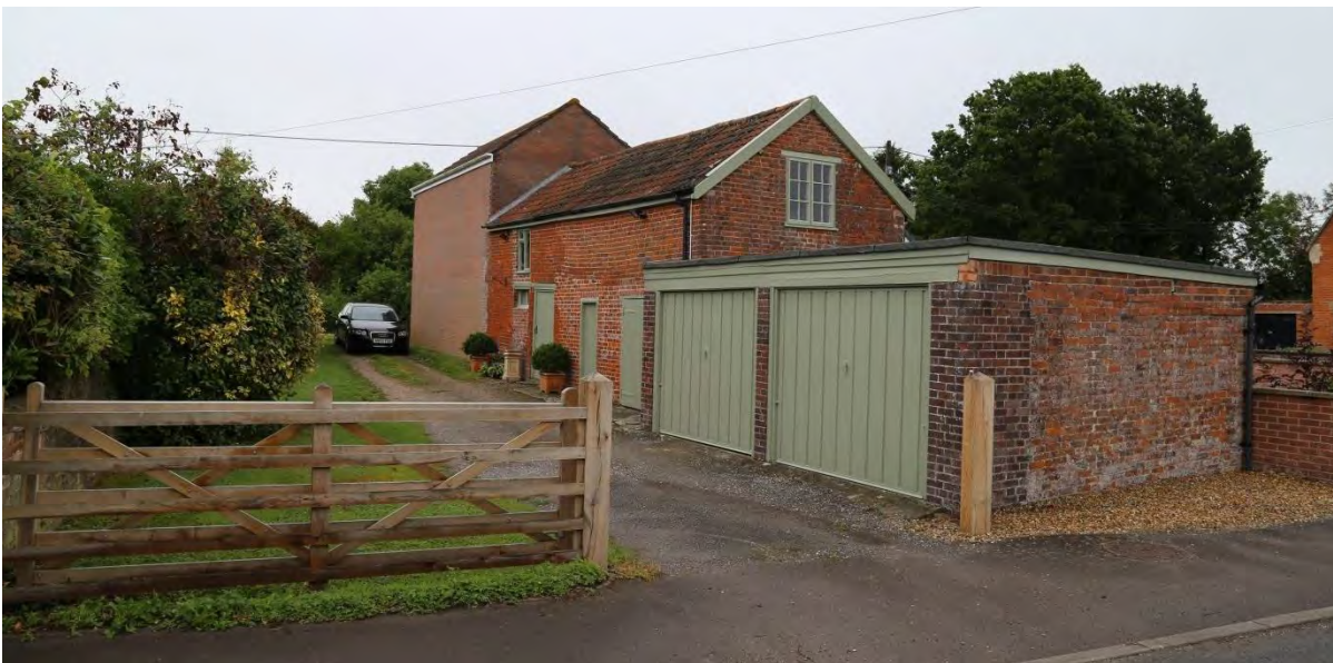
Restored property and outbuilding, Foster's Hill:
