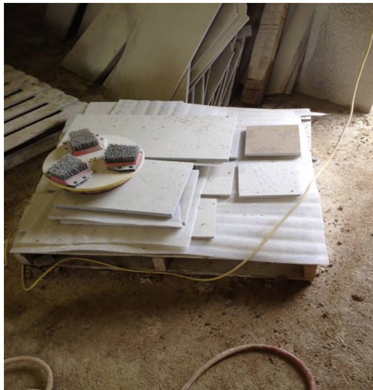
5. Cut tiles ready for polishing
