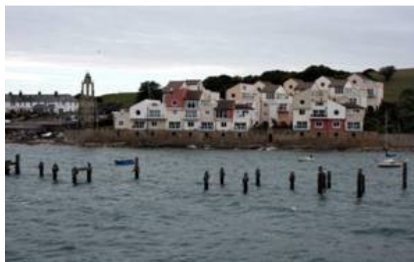
Figure 35: The Haven, a 1980s apartment development.
