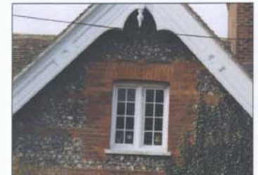
Overhanging roofs and set back windows are considered to give 'substance' to a building
