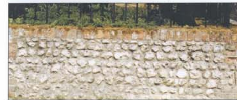
Walls with bands of flint and brick
