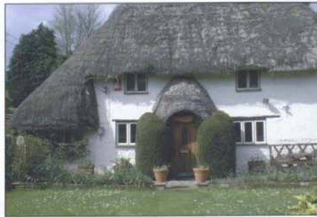
Rendered and colour-washed walls
