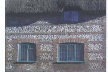
Walls with bands of flint and brick
