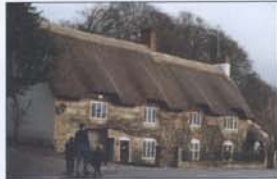
Brick and flint with thatched roof
