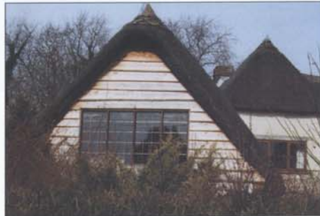
Weatherboarding and thatched roof
