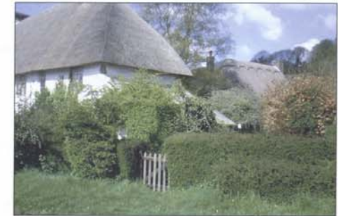
Thatched roof on cob walls
