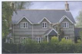
Brick and flint with slate roof
