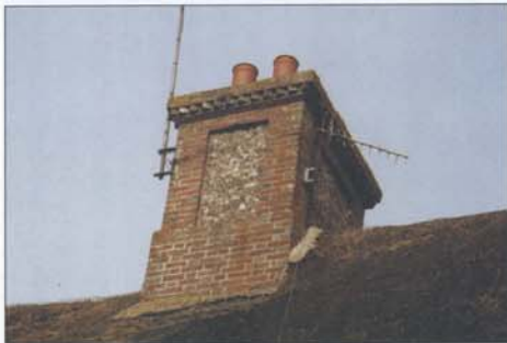
Brick and flint chimney and thatched roof
