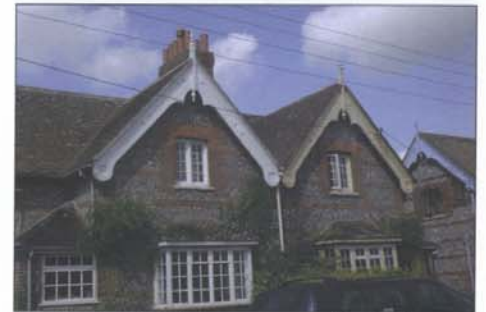
Prominent gable finials seen on several properties
