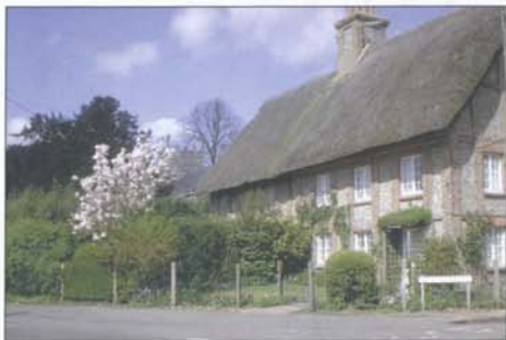
Traditional flint and brick with thatch
