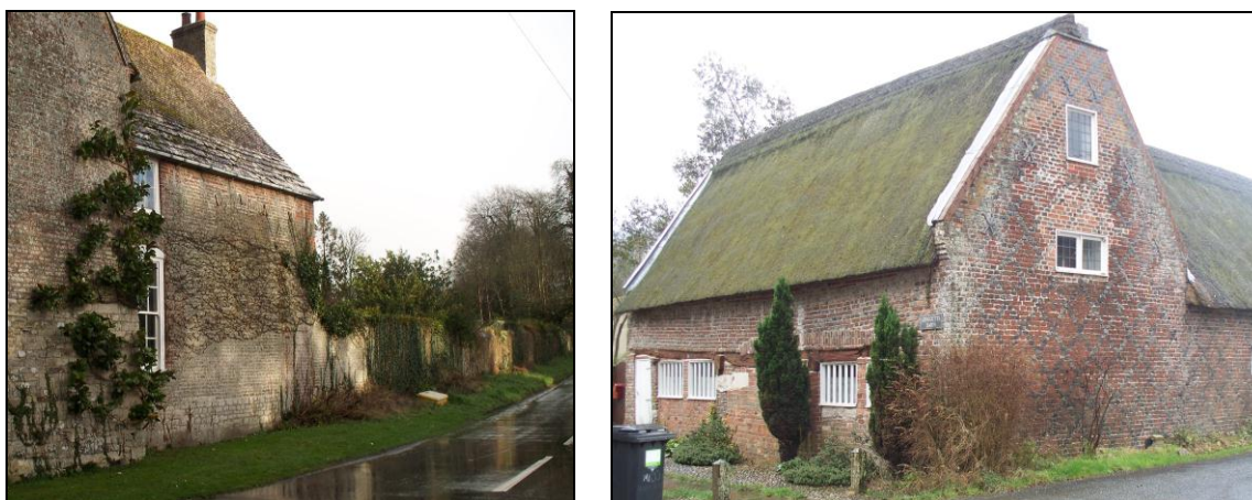
FIG. 1: Sixteenth century brickwork. Left: The rear range of the Manor House and boundary wall have both been dated to the late sixteenth century. A former brick lintel of a long blocked window is visible, showing the extent to which the building was restyled in later centuries. Extensive overgrowth by ivy and other climbers is of concern. Right: Longcutts Barn, which has decorative 'daiper' work (criss-cross pattern). The building originally had a tiled roof.
