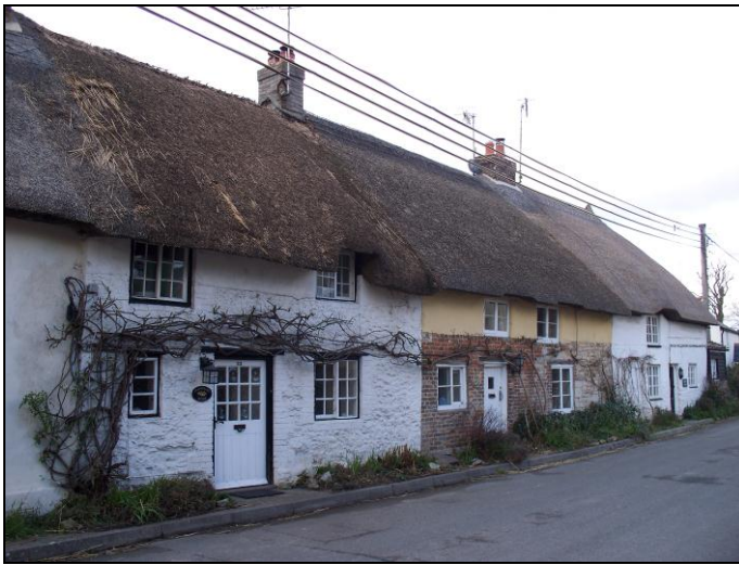
FIG. 2: Seventeenth century cottages. Nos. 20-22 originate during the period though the facades with their mixed building materials show evidence of modification over time, including possible increase from one and a half to two storeys.
