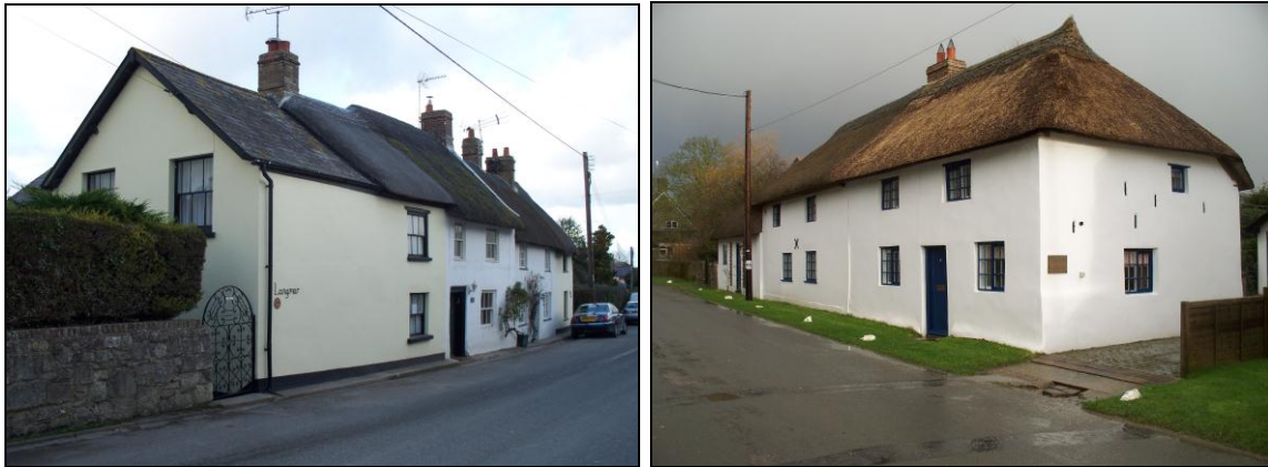
FIG. 8: Building forms along High Street. Left: Langmoor, Weston, Clovelly and Rose Lawn, a staggered terrace of cottages. Right: Badger's Thatch, Nos. 25.
