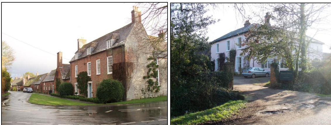
FIG. 11: Formal architectural style. Left: The Manor House (formerly Winfrith Fields Farm). One of two fine Georgian façades visible within the conservation area. Right: Marley House has seventeenth century elements, though presents a formal early/mid nineteenth century appearance.
