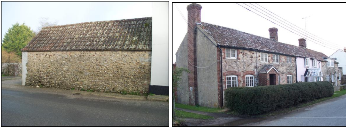
FIG. 14: Tiled roofs. Left: double Roman tiles used at Sunbeam Cottage where photographic evidence suggests they may have replaced thatch. Right: pantiles used on the roofs of Nos. 6-8 High Street. Note, in both examples walls here appear to have been partially stripped of the original protective render finish exposing poor quality rubble.
