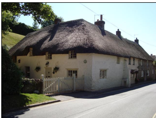
FIG. 3: The Old Bakery and adjacent cottages. The buildings have origins in the seventeenth century though were subsequently altered and extended.
