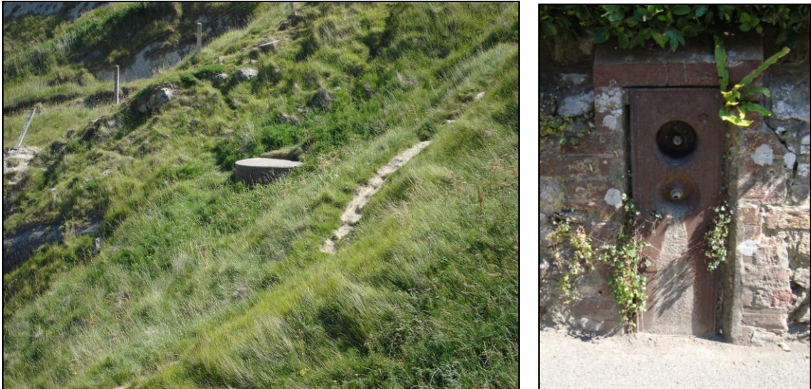
FIG. 18: Features of interest. Left: cylindrical concrete pillbox concealed on the west side of the Cove. Right: old water tap.
