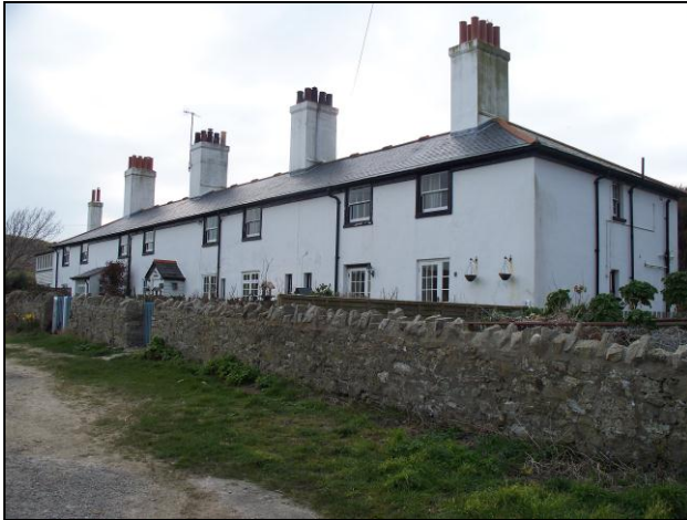
FIG. 16: Coastguard Cottages. The towering chimney stacks are the most distinctive feature of the building, their presence emphasised by the relatively shallow pitch of the roof. Modern vents set in the ridge are a visual distraction.
