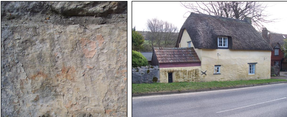
FIG. 14: Limewash. Left: traces of historic limewash finish at No. 12 Main Road. Right: renewed limewash finish at No. 7 Main Road – a building whose roof has clearly been raised (see render line with traces the original eaves level).
