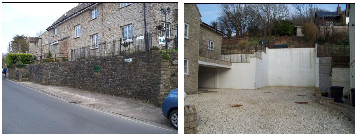
FIG. 10: The negative visual impact of retaining walls and pulling in spaces.
