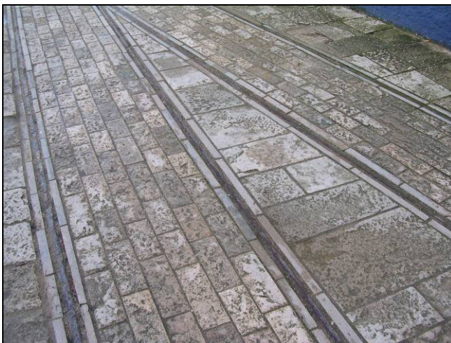
FIG. 25: Tramway rails. Now set within stone paving.
