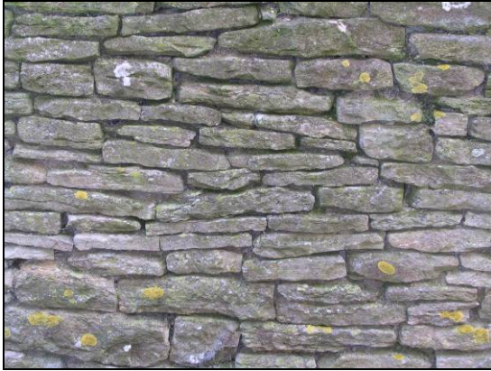
(a) Early stonework. Narrow coursed rubble. Pointing originally flush.
