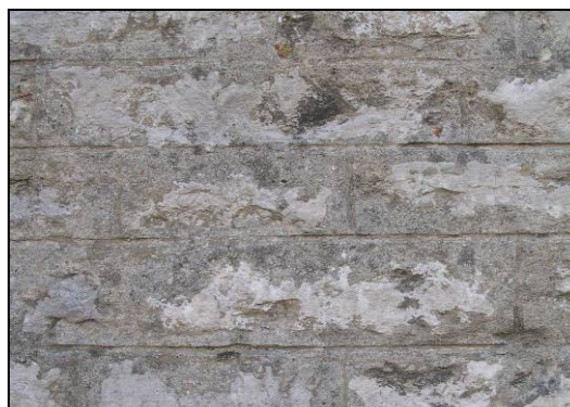
FIG. 44: Inappropriate repointing. Raised strap pointing in hard cement mortar accelerates erosion of the stone surface (seen right) and looks ugly. Buttered pointing crudely lined out (below) is also incorrect. A flush pointing on stonework using non-hydraulic lime mortar coloured with stone dust is more traditional.
