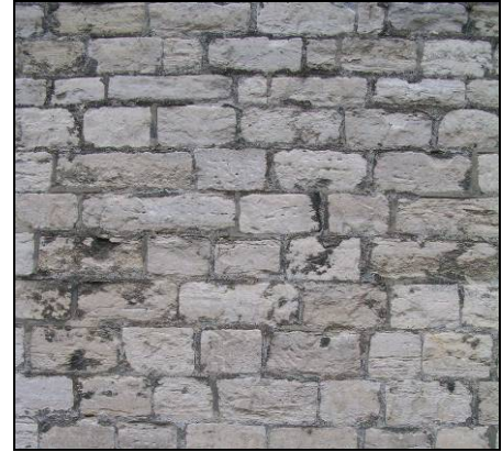
(b) Georgian. Coursed squared rubble. Faces dressed. Flush pointing.
