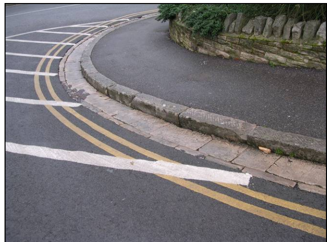
FIG. 30: Stone-lined gutters. These once occurred more widely in Swanage, and others can be viewed on Court Hill in Zone 1.
