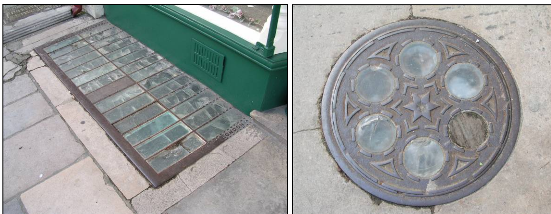
FIG. 20: Groundscape. Left: pavement light prior to being smothered with cement (see FIG. 45). Right: combination pavement light/coal hole outside the Town Hall.
