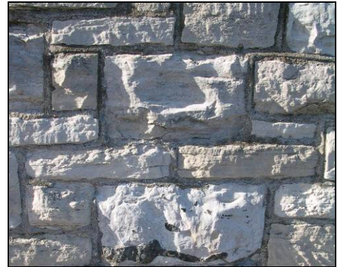
(d) Late Victorian. Neatly squared rock-faced blocks randomly laid. Irregular sizes. Flush pointing.
