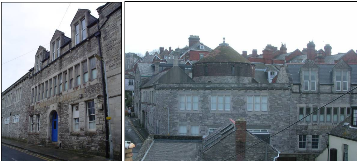
FIG. 37: George Burt's Water and Gas buildings. Left: façade on Marshall Row. Note painted sign which indicates later Masonic use of the building. Right: view of the water tower and Sentry Road elevation from Mowlem's observatory. Roofs and chimneys of Park Road are visible in the background.
