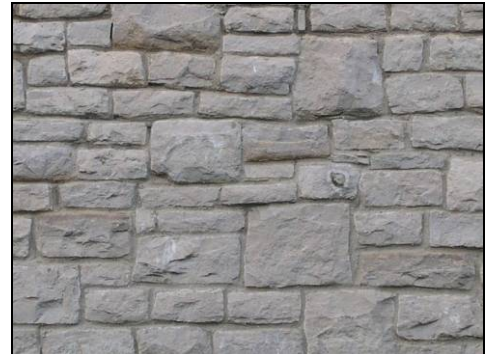
(f) Modern cladding. Randomly laid, coarsely squared rubble in irregular sizes. Recessed pointing.
