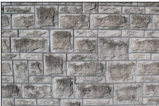
(e) Modern cladding. Random machine cut rock-faced stone in irregular sizes.
