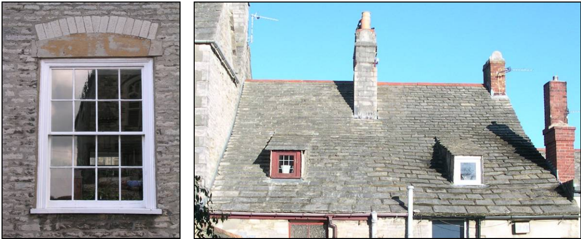
FIG. 7: Window styles. Left: eight-over-eight with exposed case and without 'horns'. Note narrow glazing bars and reflective qualities of antique glass. Right: small tunnel-like dormers to the rear of 209/211 High Street.
