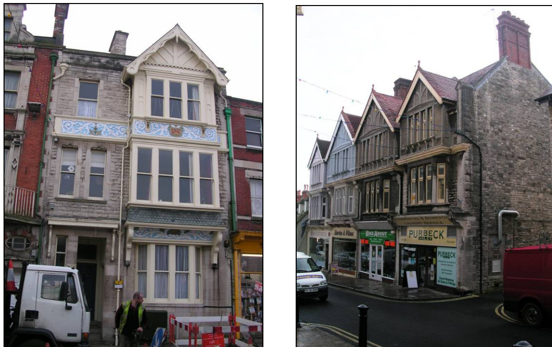
FIG. 23: Arts and Crafts inspired design on the High Street. Left: 45 High Street. Right: 67-73 High Street. Facades are virtually intact and show typical use of gables, timber cladding and pargetting. A vent pipe disfigures No.73.
