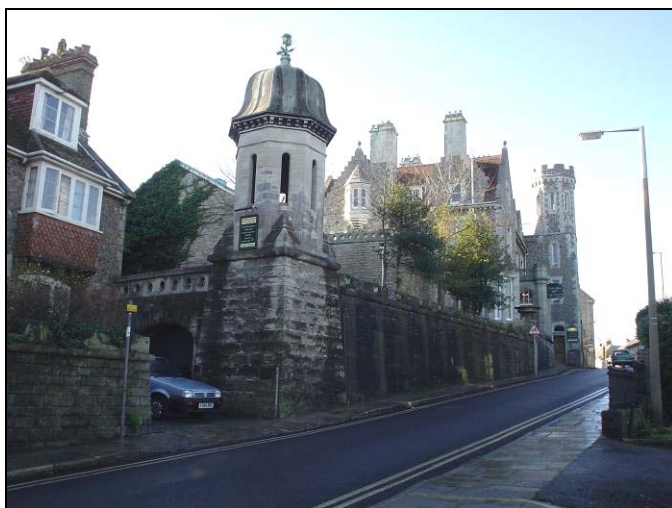
FIG. 19: View of Purbeck House up the High Street.
