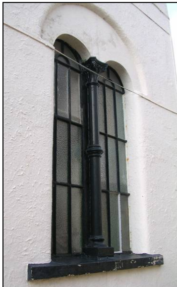
FIG. 14: Window forms and styles. Left: Romanesque style iron framed window with cast iron baluster. Centre: sash windows with margin lights on the upper panels. Ornamented dormer. Right: corner oriel with cupola on Mermond Place.
