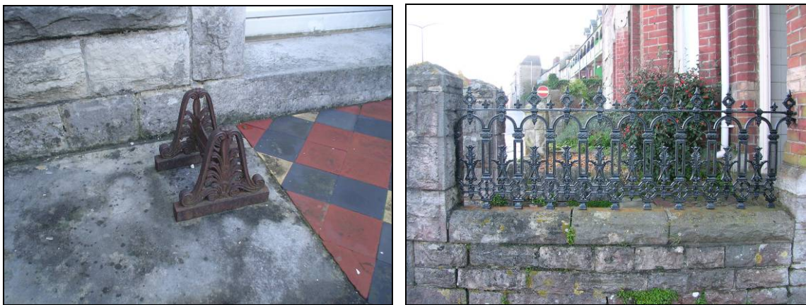
FIG. 8: Historic Ironwork. Left: acanthus leaf bootscraper at 126 High Street. Right: cast iron railing panel 257 High Street.
