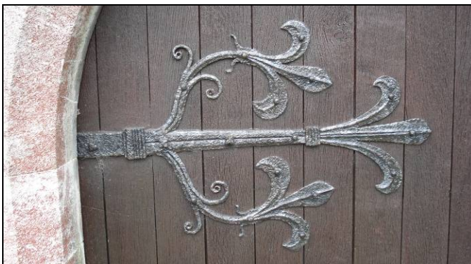
FIG. 9: Ironwork. Below: ornamental hinge at St. James'. The fine detail has been damaged by a combination of corrosion and thick brown paint. Right: tap set in the mouth of a lion's head in South Street.
