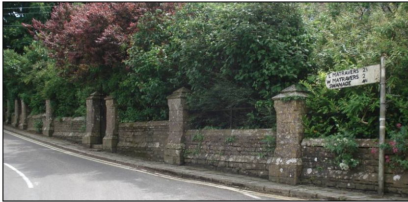
FIG. 5: Enclosure. Except where subject to damaging breaches, stone walls strongly demarcate public and private space. This run of wall with rail belonging to the old school is a prominent feature upon entering the village.
