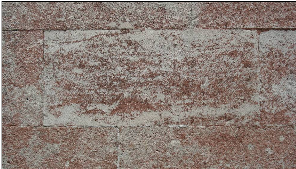
FIG. 10: Stonework at St. James'. The finely tooled surface of the fine ashlar blocks has been extensively colonised by red lichen.
