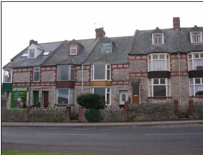
FIG. 12: Brick detailing on stone. The combination of local stone with dark red Swanage brick is particularly characteristic of late nineteenth century development in and around Swanage. Note the range of unattractive alterations to windows, doors and roofs that have taken place.
