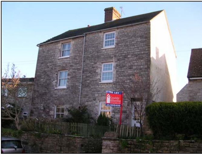
FIG. 6: Poor window design. The house on the right has had its windows replaced. Manifestly plastic, their flat detailing is obviously superficial and the proportions used irregular and thick. Top opening they lack the profile of a sash window, while their 'Georgian' configuration has been applied to what is probably a Victorian building.
