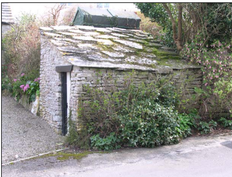
FIG. 2: Rustic outbuilding. The heavy roof of rough-cut slabs is similar to the vernacular structures erected around quarry heads in Purbeck. Similar buildings survive in several locations around Herston.
