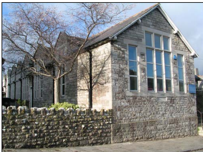
FIG. 9: St. Mark's CofE School, Bell Street. The older part of the school has a bold presence. It is unfortunate that plastic windows have been installed.
