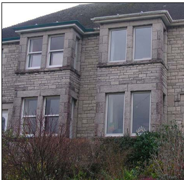
FIG. 15: Window contrasts. Sash windows have here been replaced with blank panels which give an uncharacteristically strong vertical emphasis and blandness to the facade.
