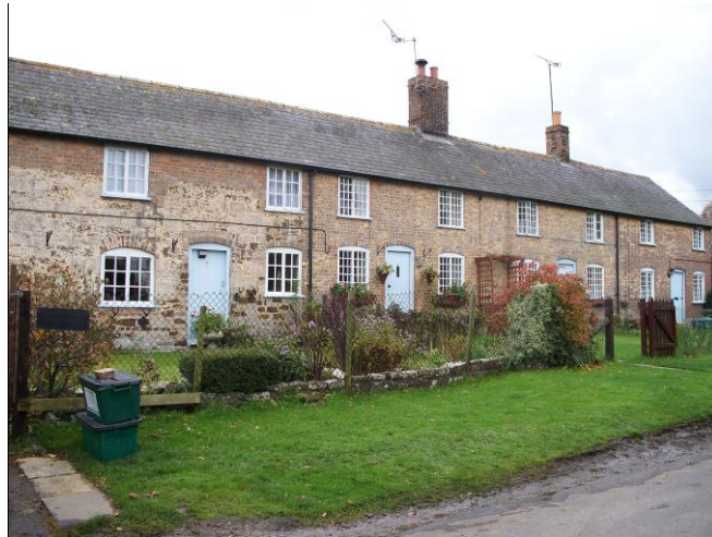
FIG. 10: East Holme Cottages. No. 1 to the left incorporates heathstone in its construction, though the terrace is otherwise built using a buff brick. The terrace appears to have been limewashed in the past.
