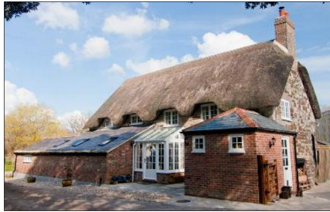
FIG. 11: Priory Farmhouse. An eighteenth century building, possibly incorporating materials derived from former monastic structures, this is one of only two thatched buildings in the village. The walls of the cottage are heathstone, with later brick additions which greatly obscure the frontage.
