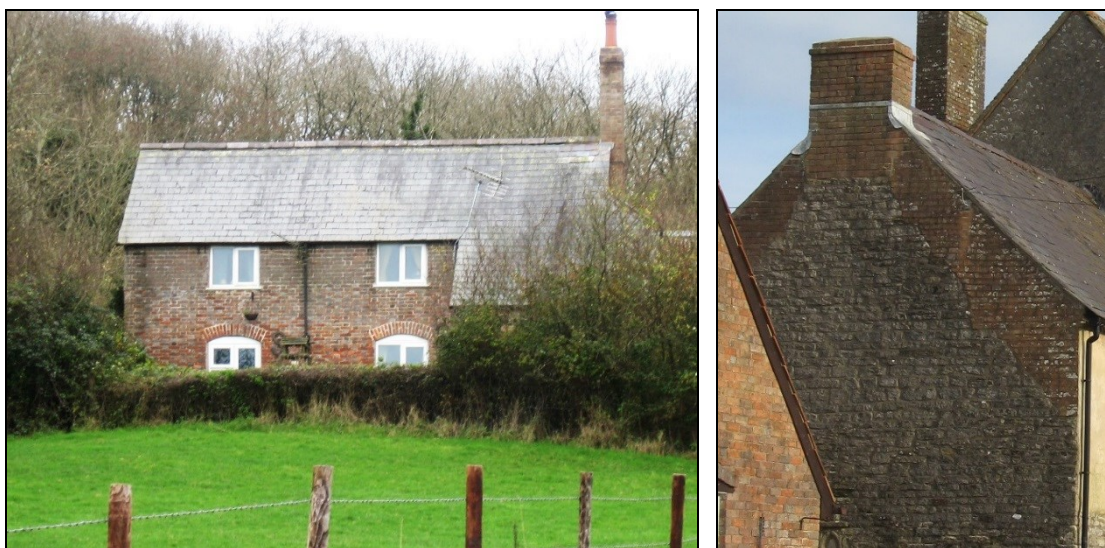
FIG. 5: Increases in height. Both Keeper's Cottage (left) and the west side of East Creech Farm (right) show signs of a historic increase in height. At Keeper's Cottage the band of brickwork at first floor level is a different colour to that below, whilst brick has similarly been added above stone at the farmhouse. Each carries a slate roof though given the age of the buildings the original coverings would have been different. Keeper's Cottage may have originally been a single storey thatched dwelling.
