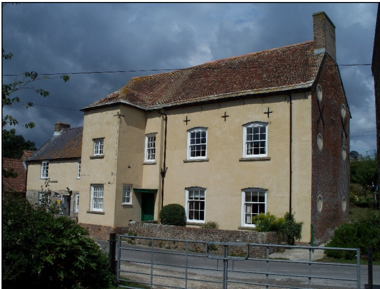
FIG. 7: East Creech Farmhouse. The west half of the building (also see cover photo) dates to the seventeenth century and has been increased in height, whilst the east range appears to have been more substantially remodelled during the eighteenth century. The two storey porch is an interesting feature.
