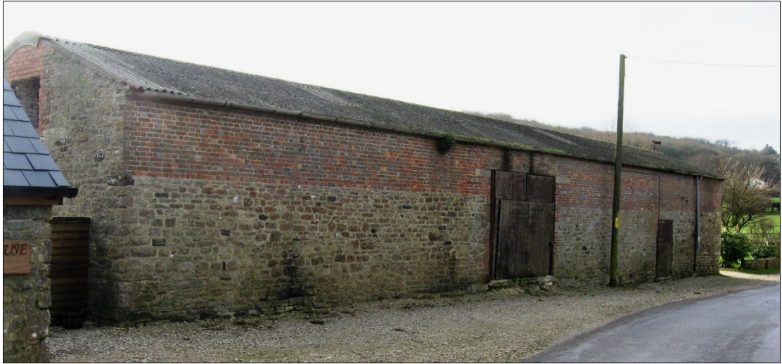
FIG. 8: Stonework. The barn opposite East Creech Farm features a mixture of limestone and heathstone rubble. The walls have been raised or modified in brick. The building was heavily altered during the twentieth century and is compromised by the sheet roof and poorly formed entrance which was previously arched.
